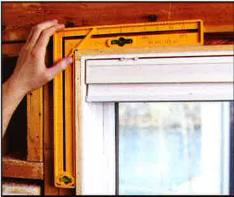
Accurately install windows and doors
